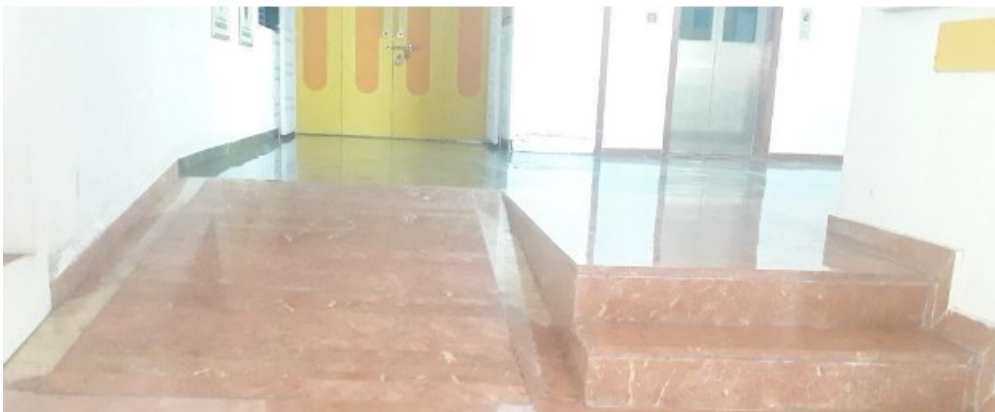
Ramp from Main lobby to lifts
