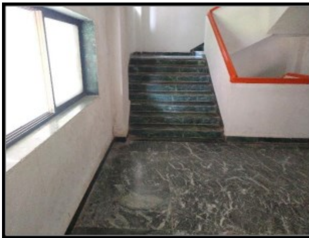
Daylight at Staircase
