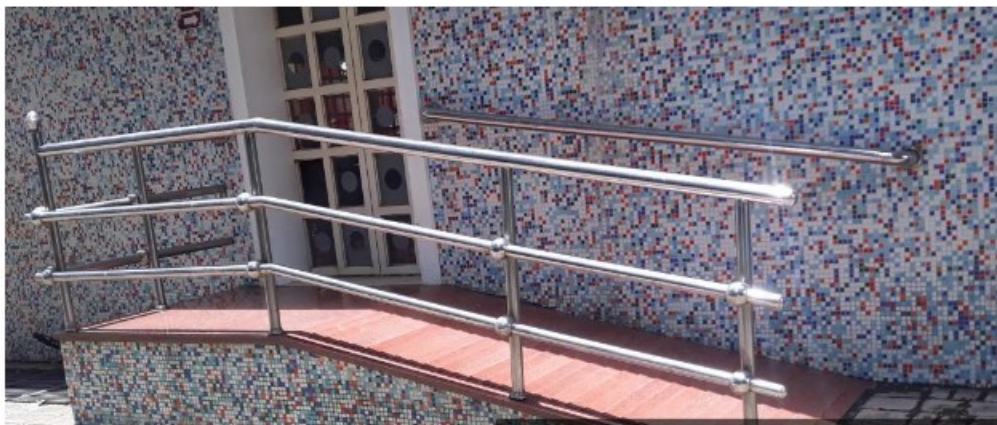
Ramp at entrance to Lobby
