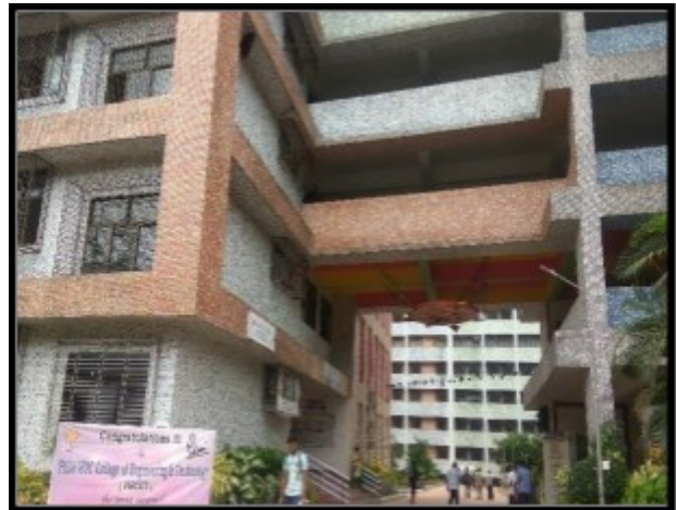
Maintenance Free tiles on the building
