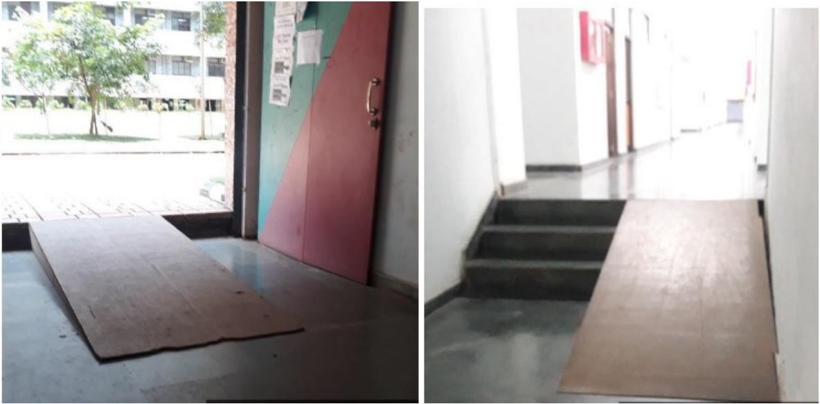
Ramp at basement and near recreation area
