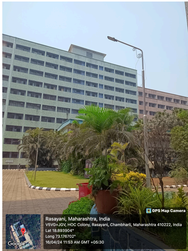
(Solar Powered Street Lamps in Campus)
