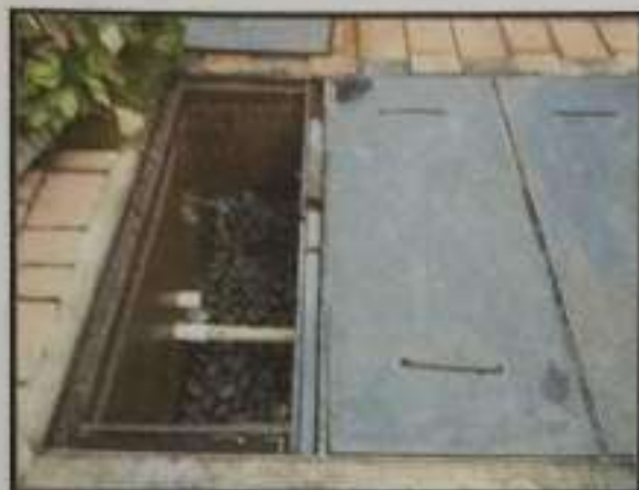
Rainwater Harvesting System- Recharge Pit
