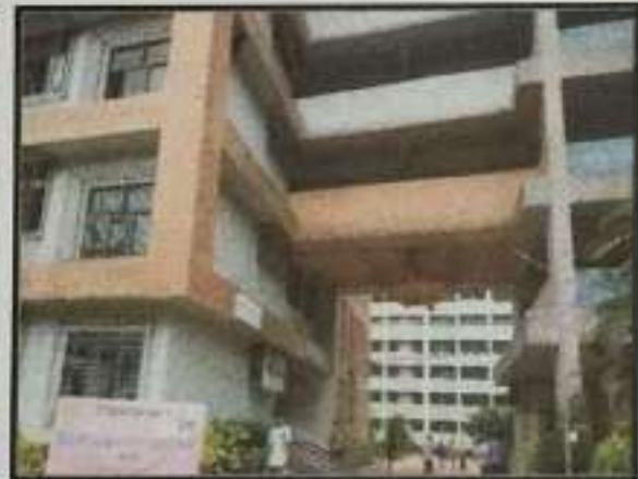
Maintenance Free tiles on the building
