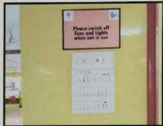
Signages near switch boards
