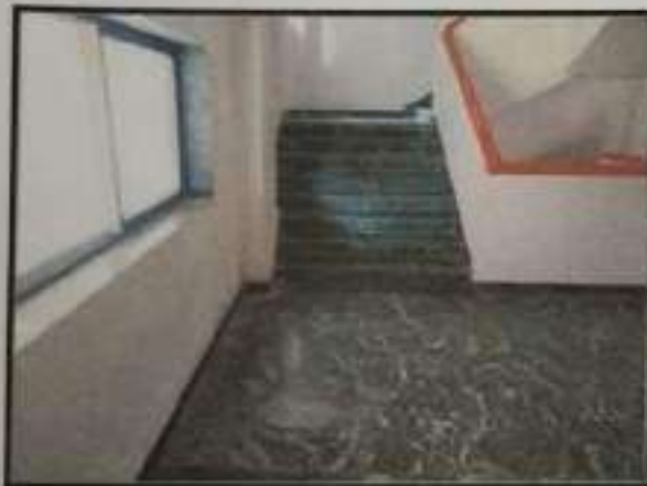
Daylight at Staircase
